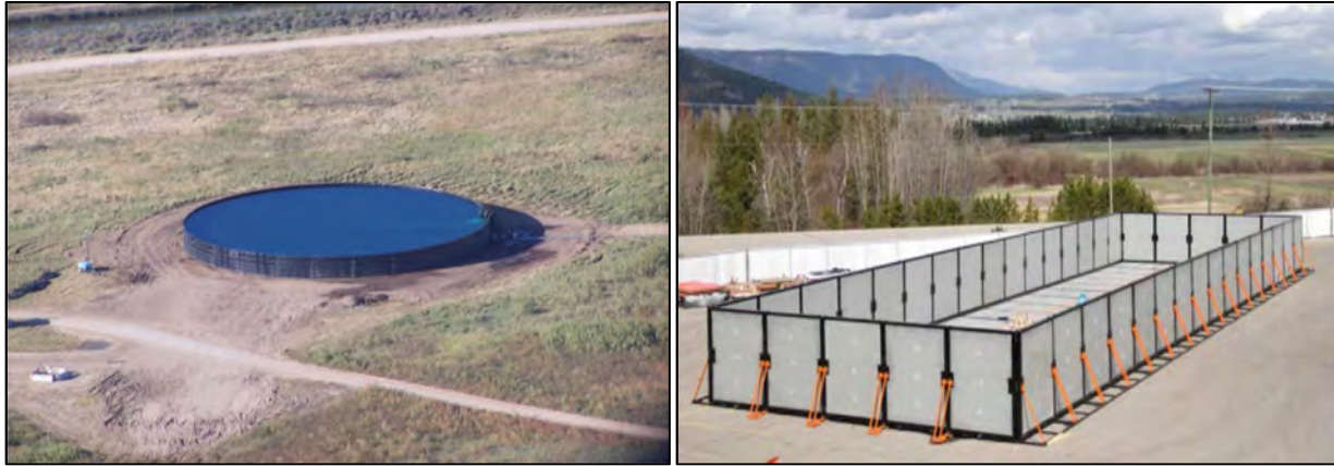
Figure 4-5: Modular Large Volume Tanks.
