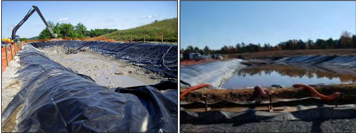
Figure 4-1: Pits with Visible Liners.
