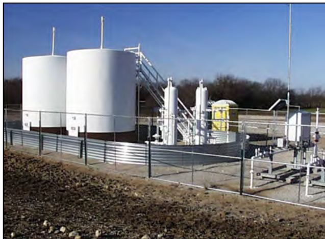
Figure 4-4: Tanks with Secondary Containment.
