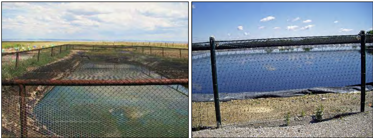
Figure 4-2: Pits with Fencing and Netting.
