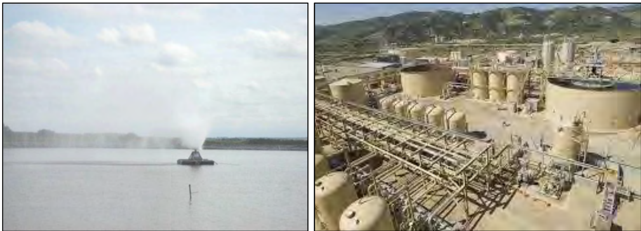
Figure 4-7: Treatment and Disposal Facilities.
