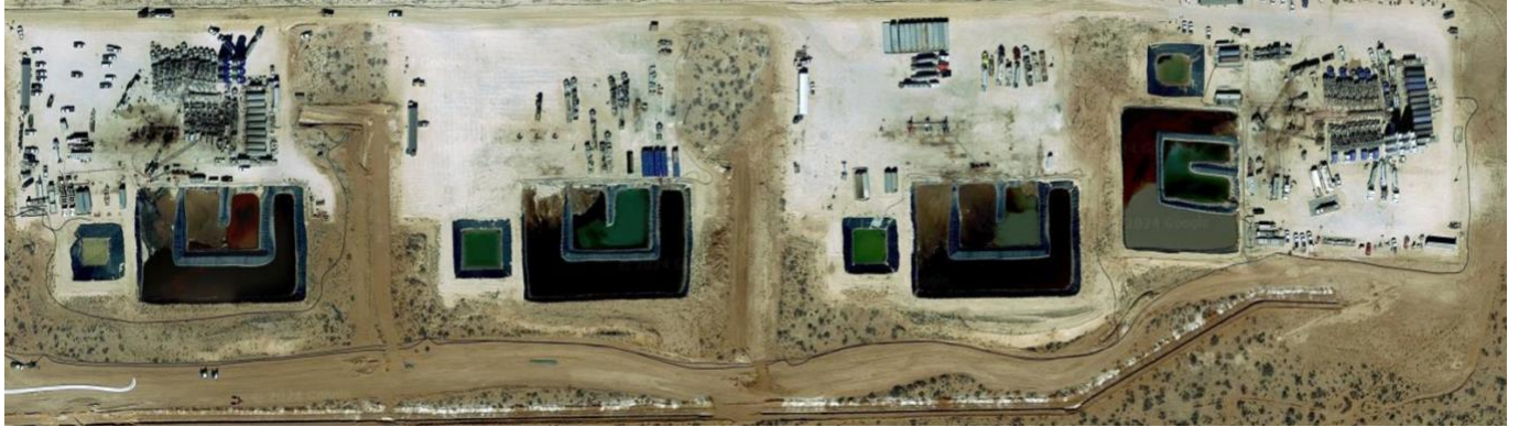
Figure 2b. Multi-Well Pad Aerial (Permian)
