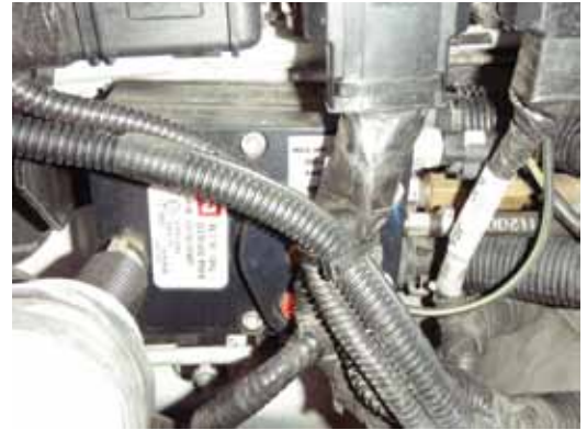
Figure 40. 2008-09 F-150 vaporizer location
