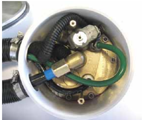
Figure 64. Later style multivalve without integrated pressure-relief valve
