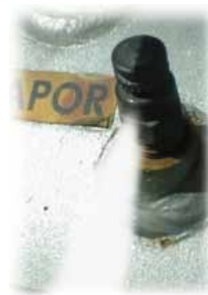
Figure 101. 80 percent fixed maximum liquid level gauge
