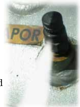
Figure 10. Fixed maximum liquid level gauge
